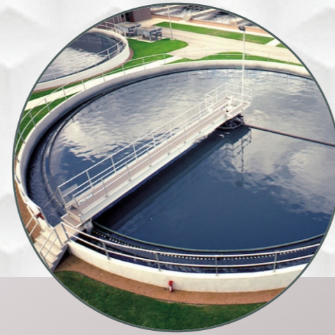
Sewerage Treatment Plant (STP)
